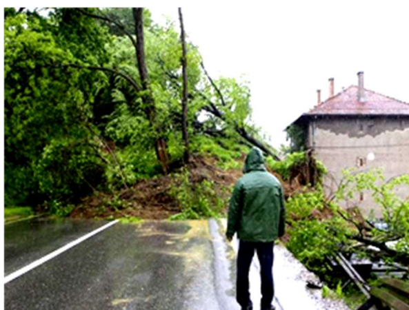
Landslide, Location: Nemila, Main road M17, Section: Topcic polje -Lasva km 3+880 (Floods 2014)
